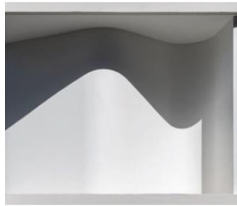
J - WHITE PAINTED CONCRETE CANDALEPAS ASSOCIATES - BOTANY ROAD
