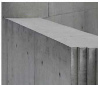
E - OFF-FORM CONCRETE CANDALEPAS ASSOCIATES - PERRY PARK
