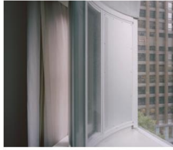
F - ALUMINIUM DOUBLE GLAZED WINDOW FRAMING CANDALEPAS ASSOCIATES - PORTER HOUSE HOTEL
