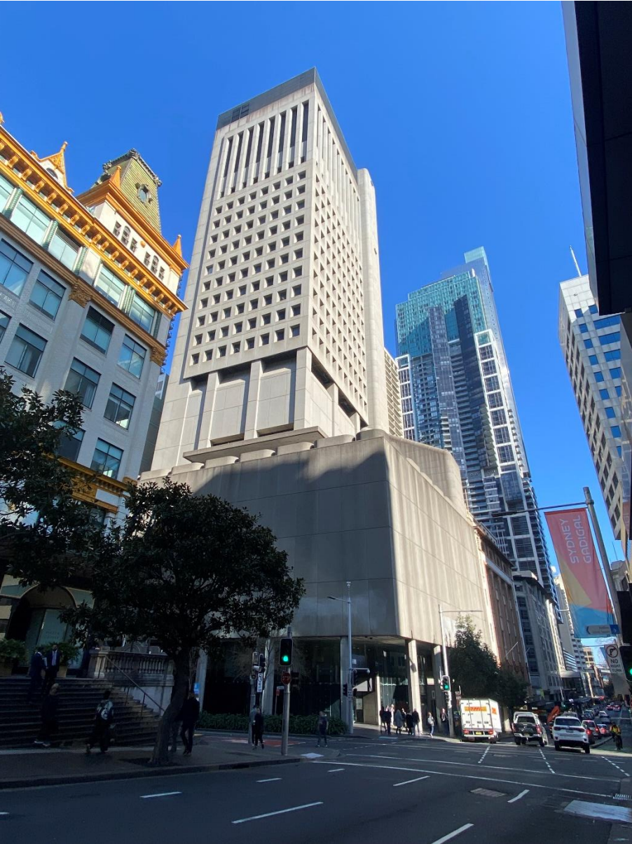
Figure 3: Site viewed looking west along Liverpool Street
